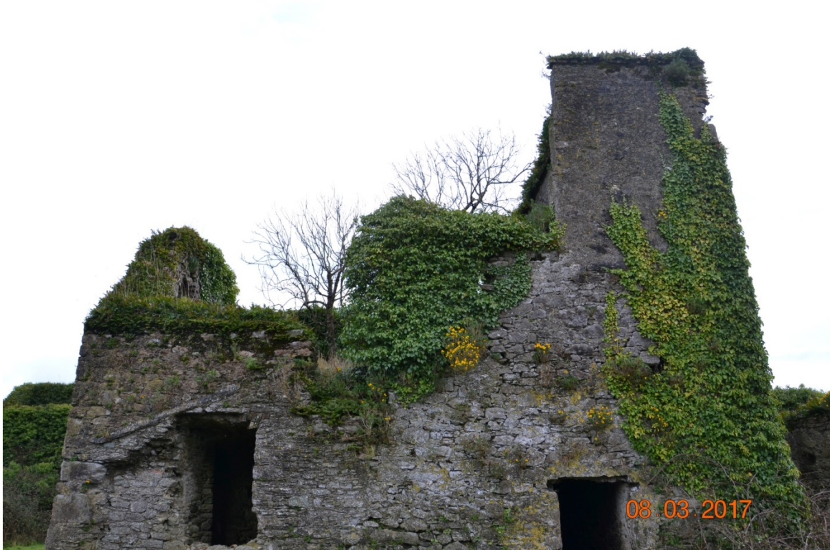
Photo 23 – View of the western elevation of the original structure on the south side.
