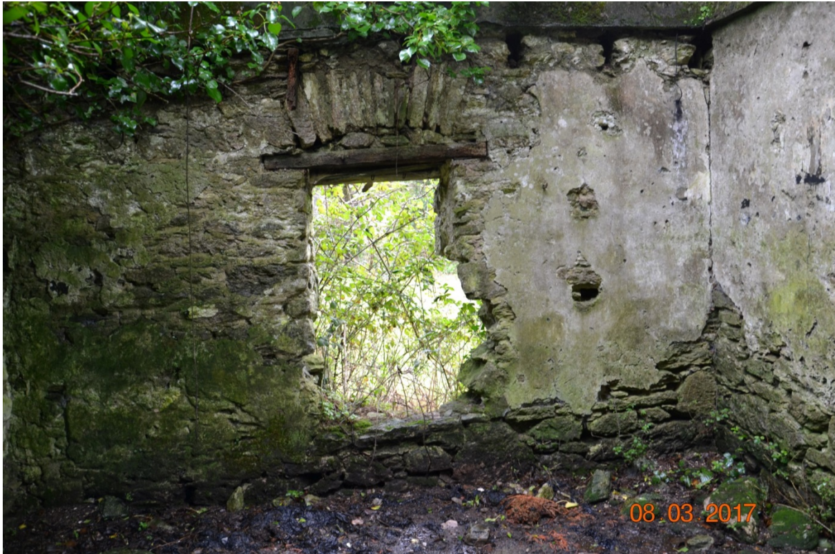
Photo 38 – Area 1. View of window ope and lintel. Looking east.
