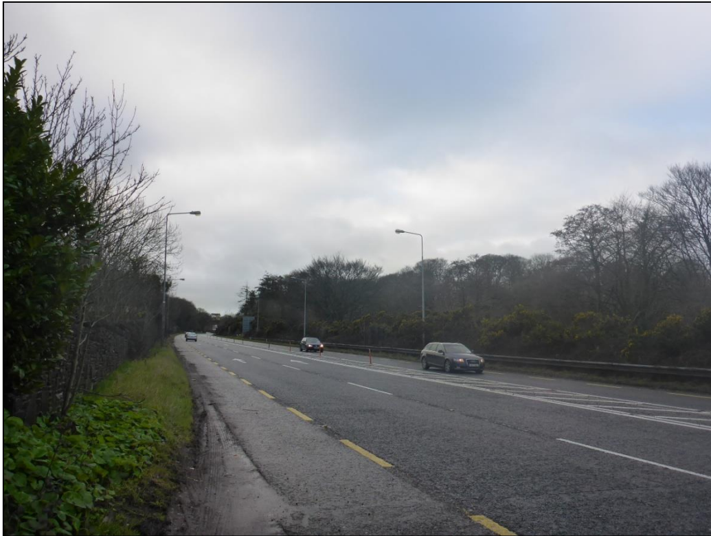
Plate 15.1 View south/southwest along existing N28 road at northern end of proposed road project, showing dense woodland boundaries (Maryborough/Mounthovel townlands)
