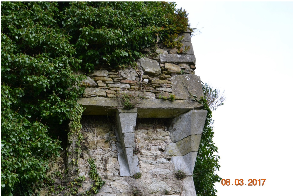
Photo 16 – View of the southern side of the bartizan.
