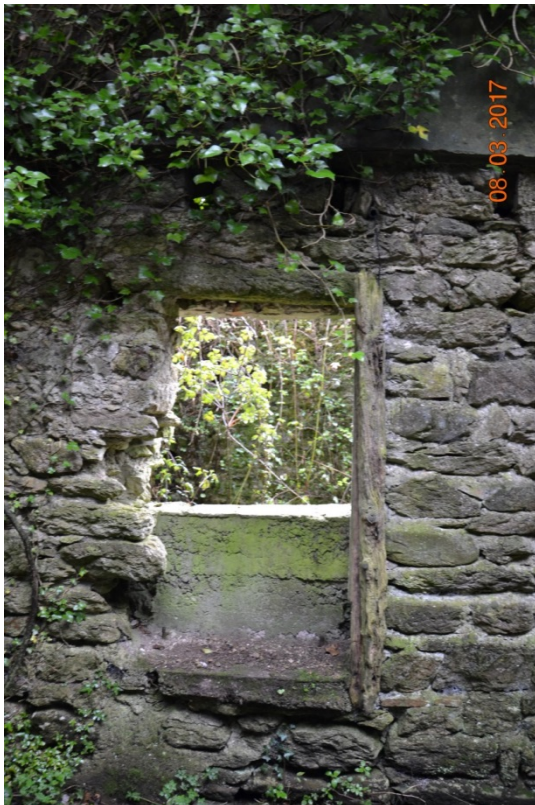
Photo 41 – Area 2. View of the window ope. Note the mass concrete fill.
