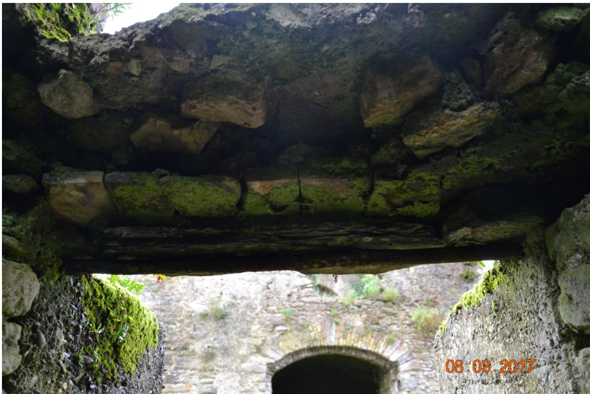
Photo 37 – Area 1. Close up view of the lintel.
