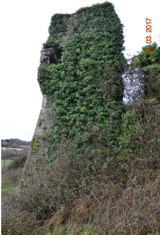
Photo 13 – View of the bartizan in the SE corner.
