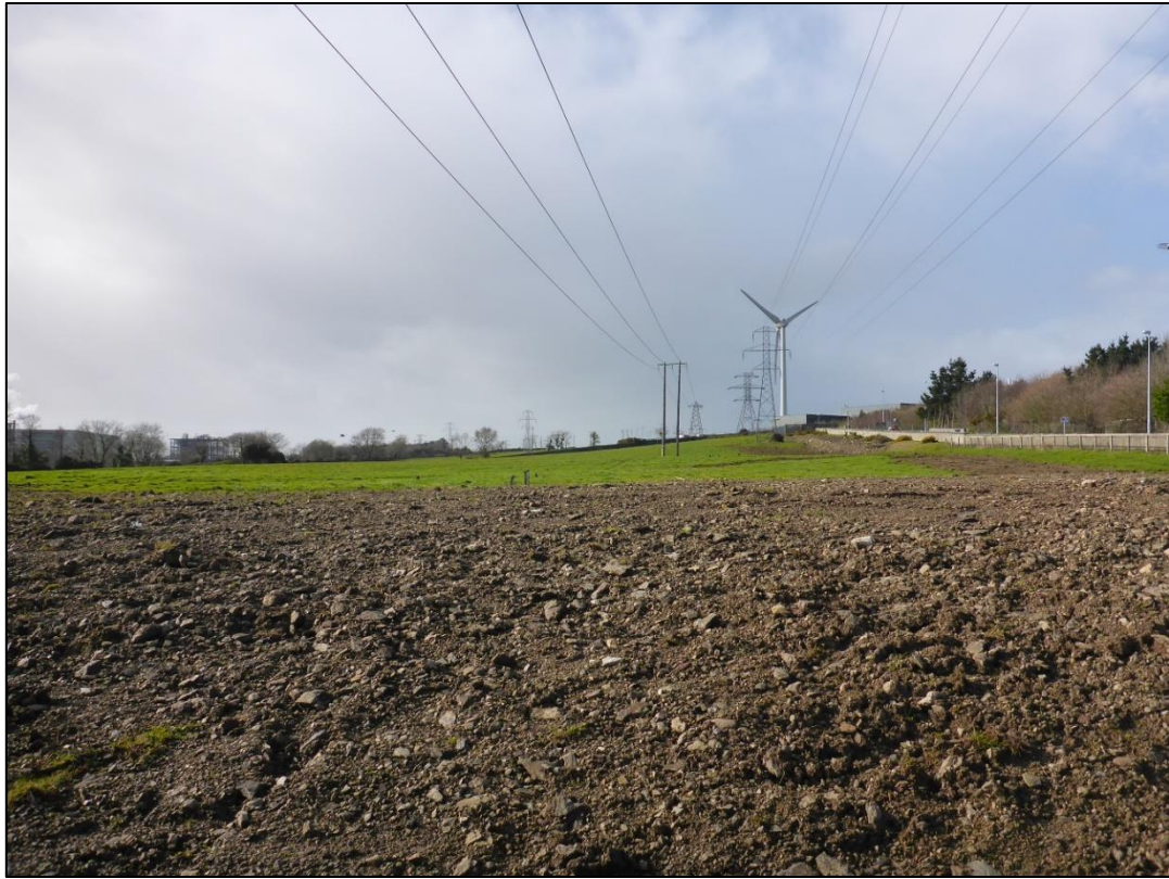
Plate 15.31 View west along proposed M28 road project in Barnahely townland (west of R613 road)
