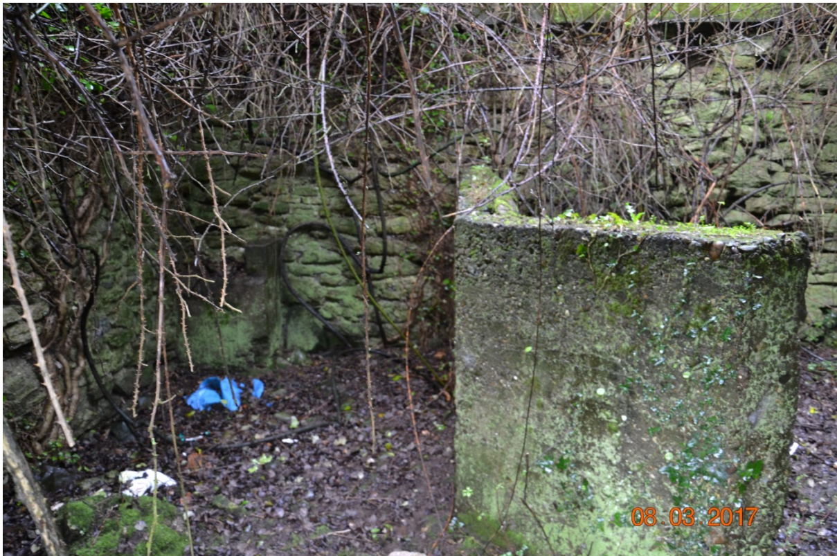
Photo 39 – Area 2. Concrete wall subdividing the space.
