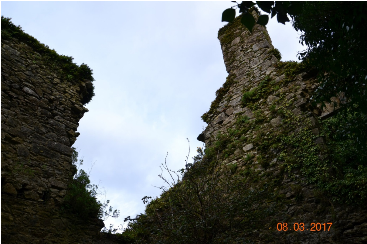
Photo 57 – Area 5. View of the northern wall, including the chimney.
