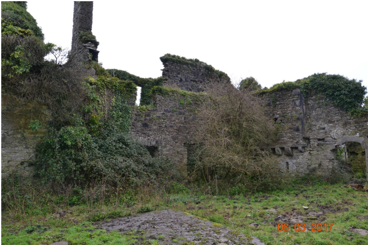
Photo 30 – View from the courtyard – from the NW.
