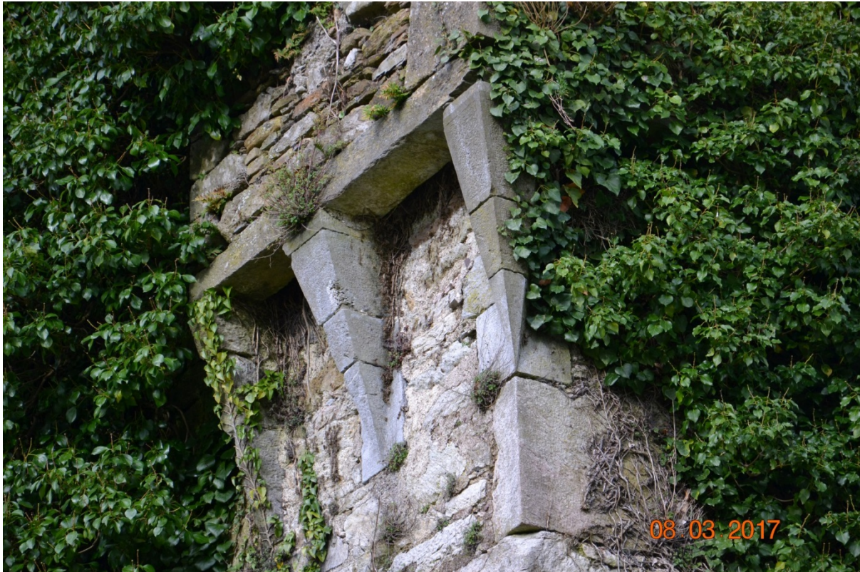
Photo 15 – Detailed stonework corbels under the bartizan. Photo from the SE.
