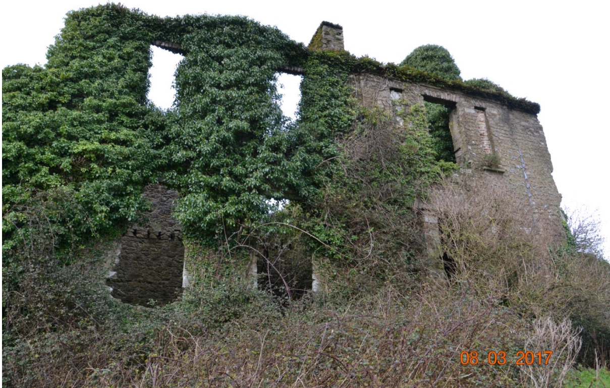
Photo 11 – View of the eastern elevation from the east.
