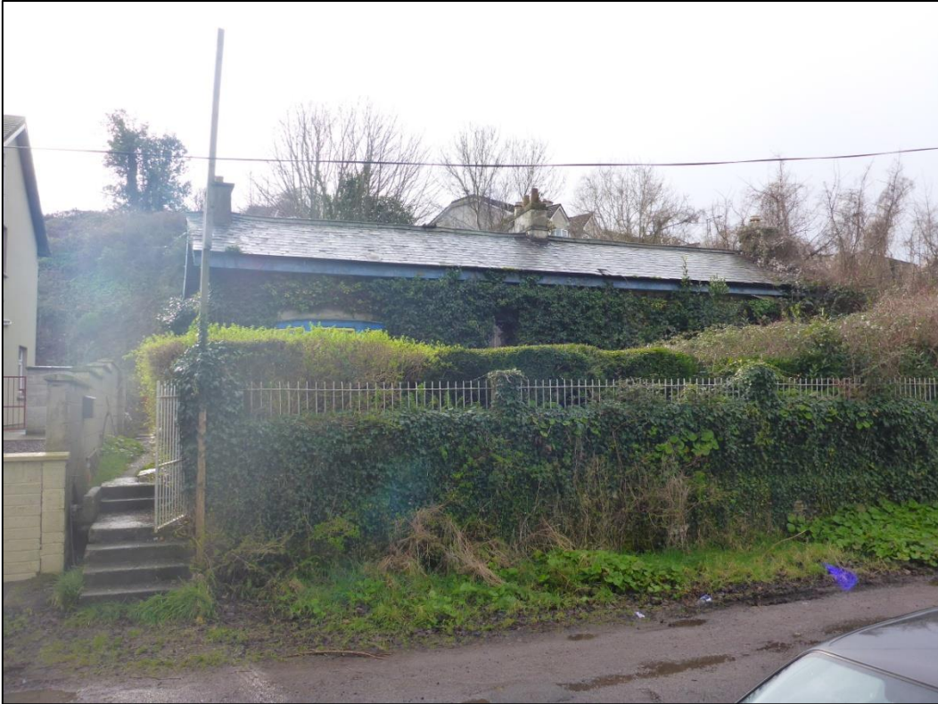
Plate 15.44 Rock Cottage (BH4) in Ringaksiddy village, facing south
