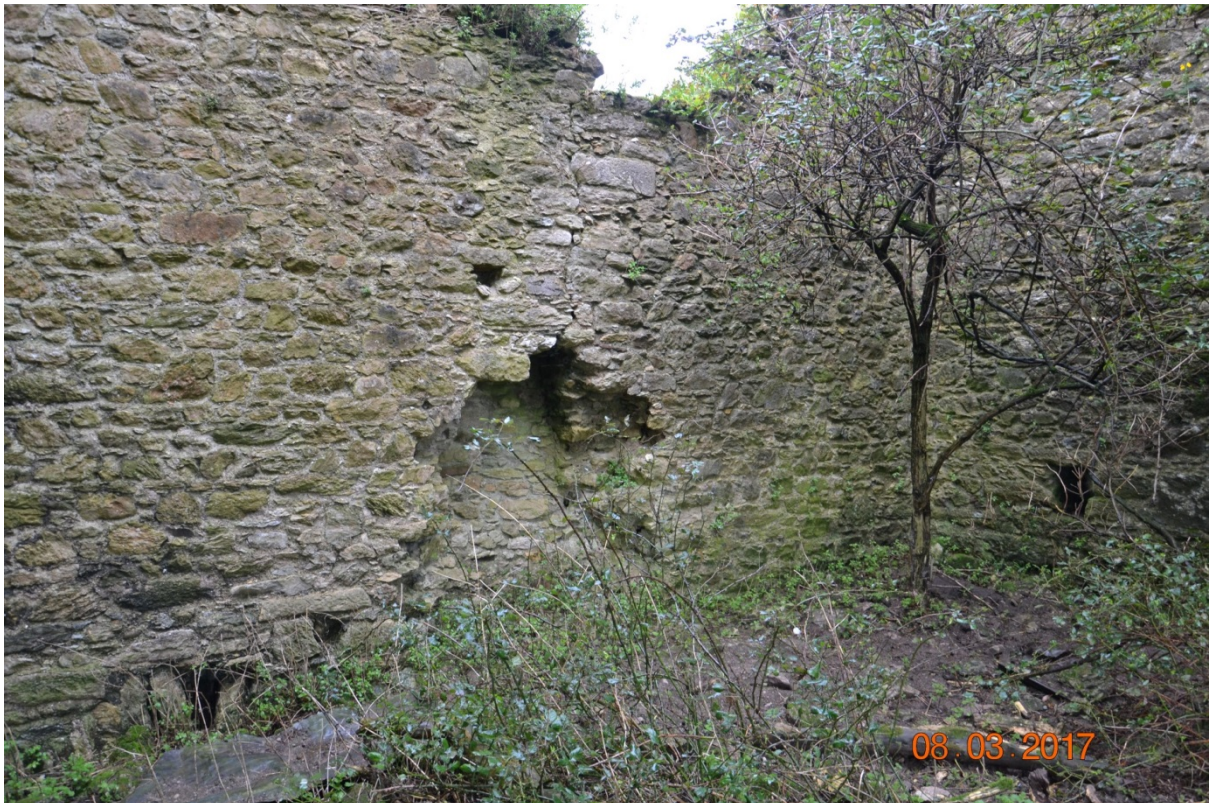
Photo 55 – Area 5. View of ope in the western wall.
