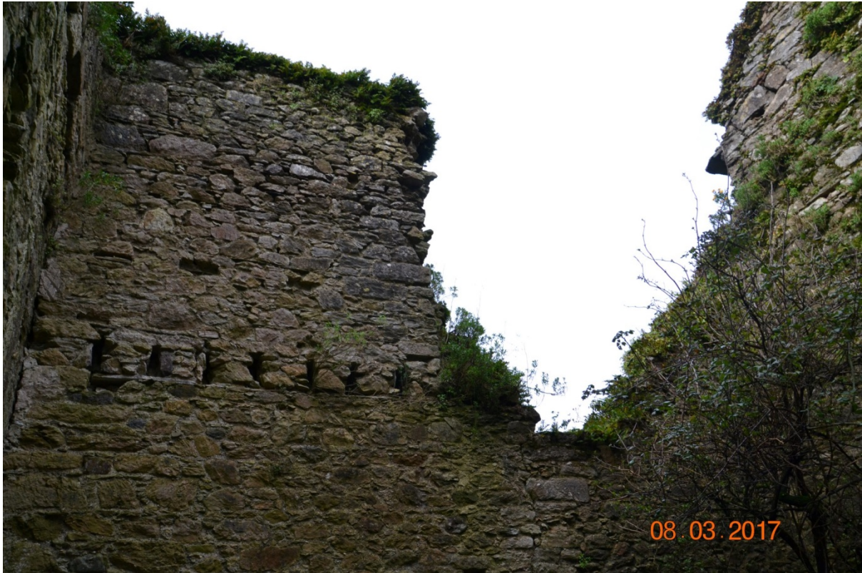
Photo 56 – Area 5. View of the upper portion of the western wall.
