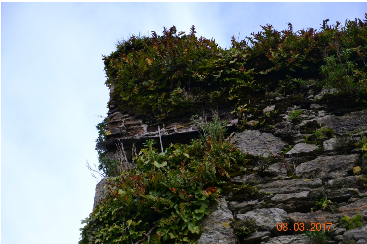
Photo 20 – Close up view of the brickwork at eaves level.
