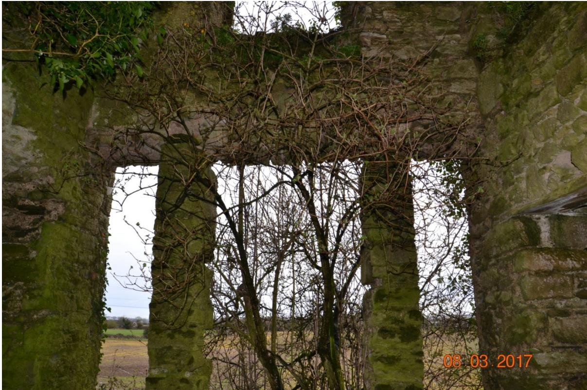
Photo 62 – Area 6. View of the lower lintels. Appear to be intact.
