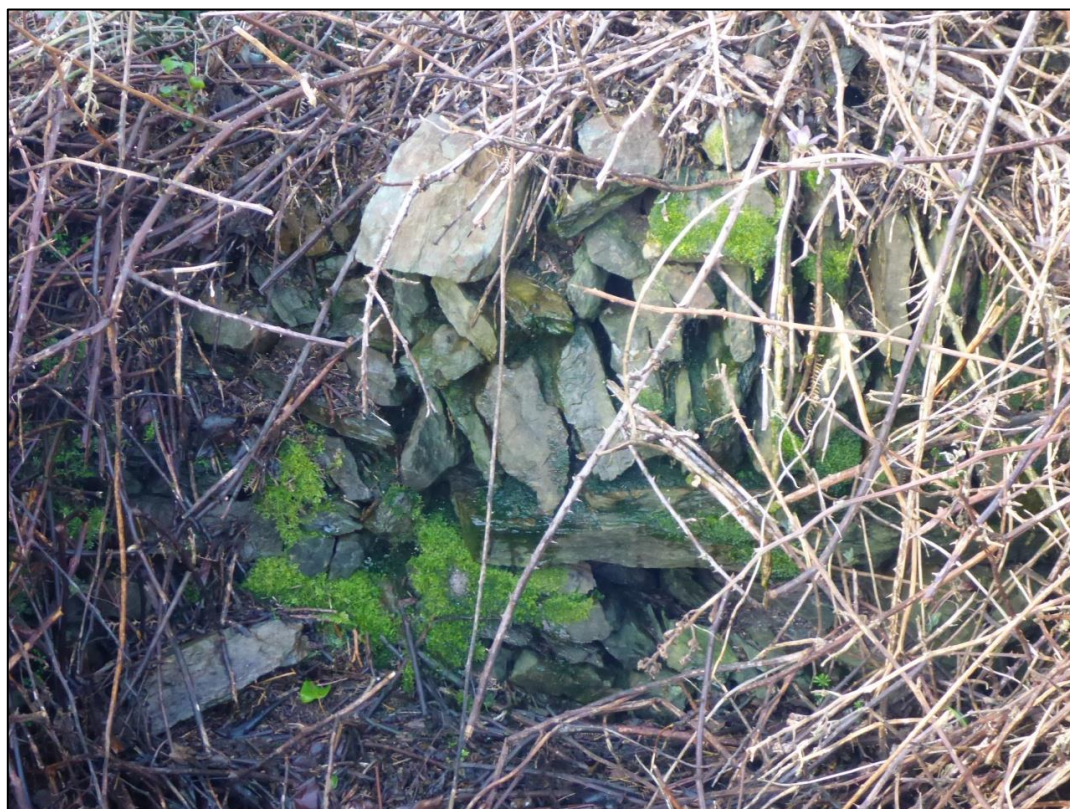
Plate 15.12 Section of dry-stone walling in field boundary (BH22), Ballinrea townland
