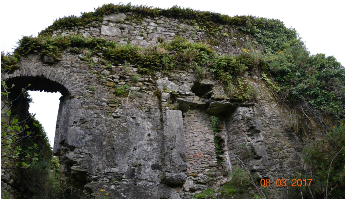
Photo 51 – Area 4. View of the upper portion of the wall.
