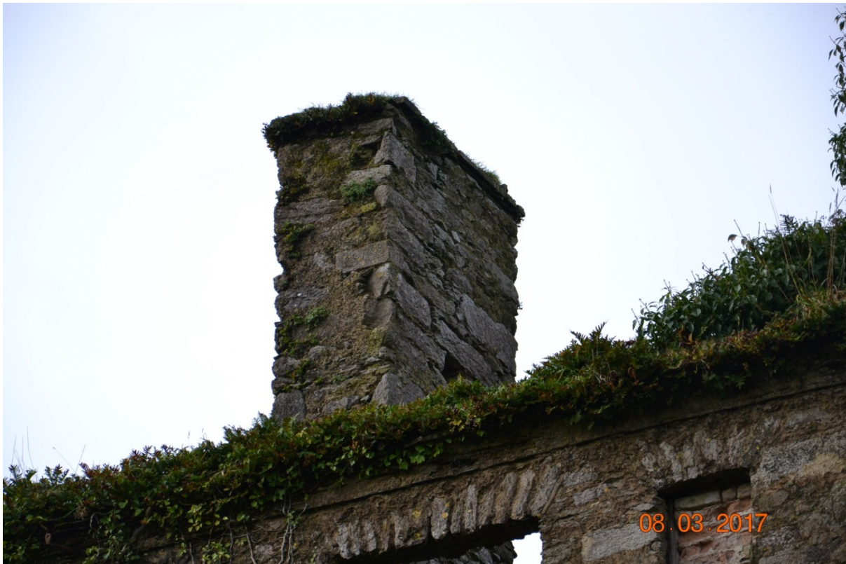
Photo 8 – View of the southern chimney – appears to be intact.
