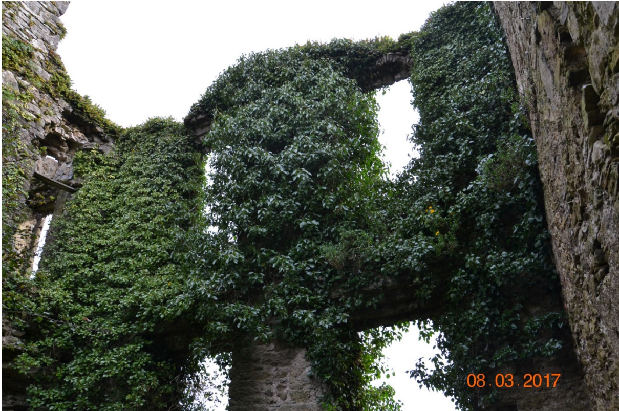
Photo 60 – Area 5. Heavy vegetation, especially at higher levels. Ope appears to be intact, but also appears to be shallow / flat.
