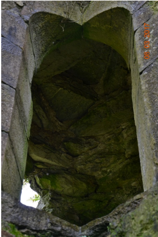
Photo 48 – Area 4. View of the roof of the bartizan.
