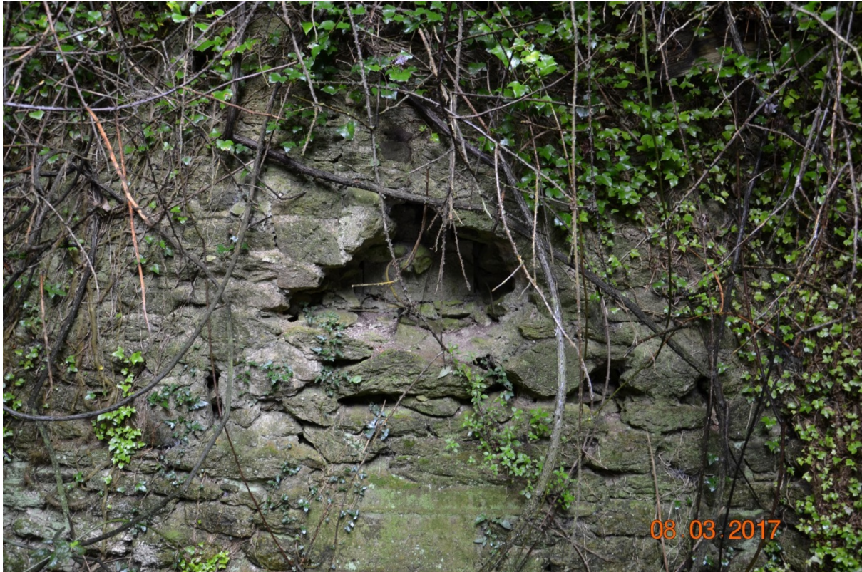
Photo 40 – Area 2 – modern concrete block in the wall.
