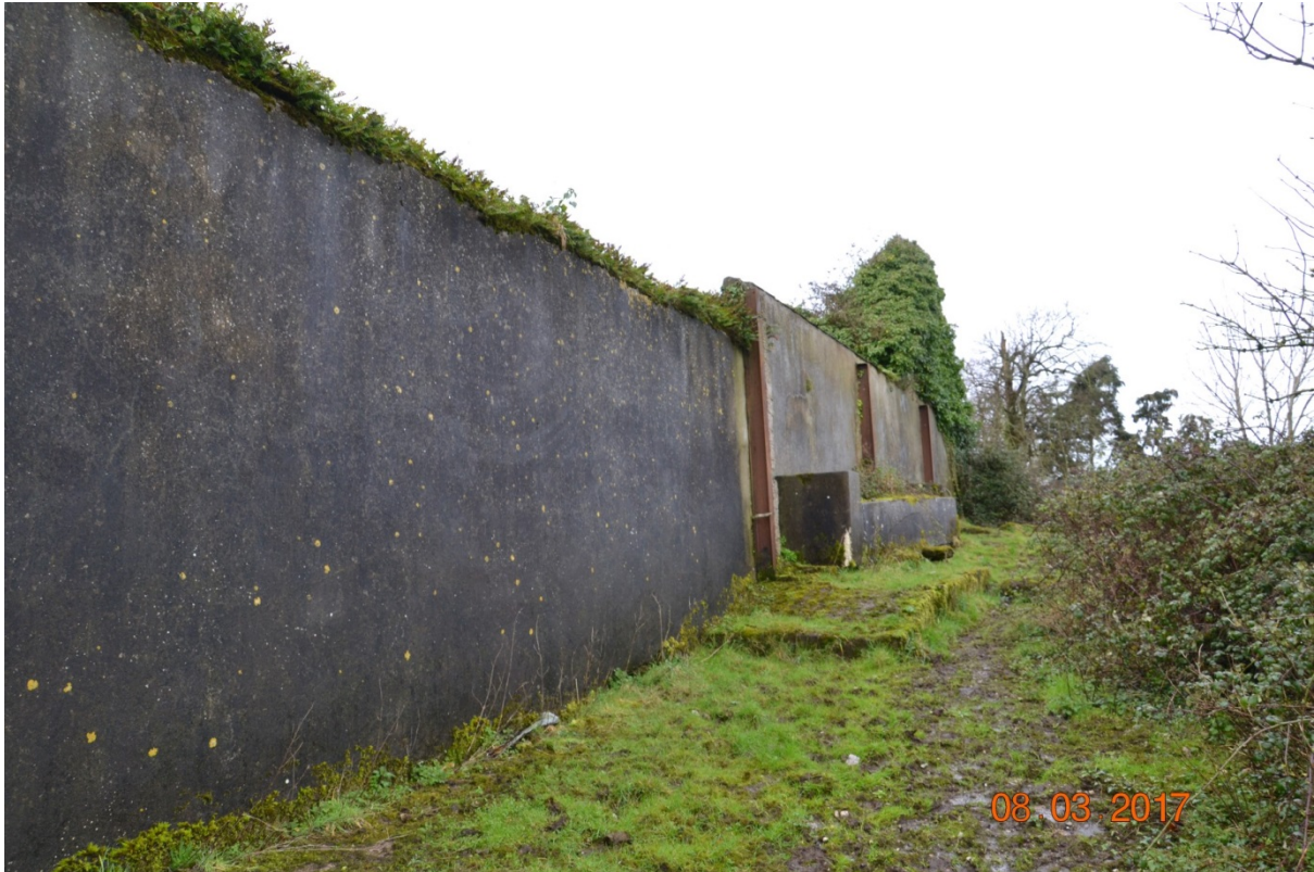
Photo 3 – View of the northern concrete wall.
